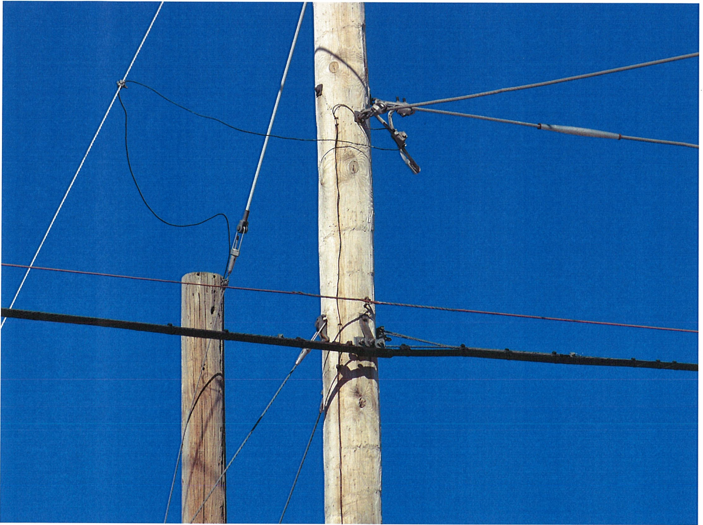
Figure 8. Close up view of CE Pole 13 is on the west side of the tracks showing all the attaching entities Fairpoint and City of Concord Fire Alarm. Note the light colored pole is the newest pole that was set in 2001 and the darker pole is the original CE Pole 13 that was set in 1967 and is now used for guying
